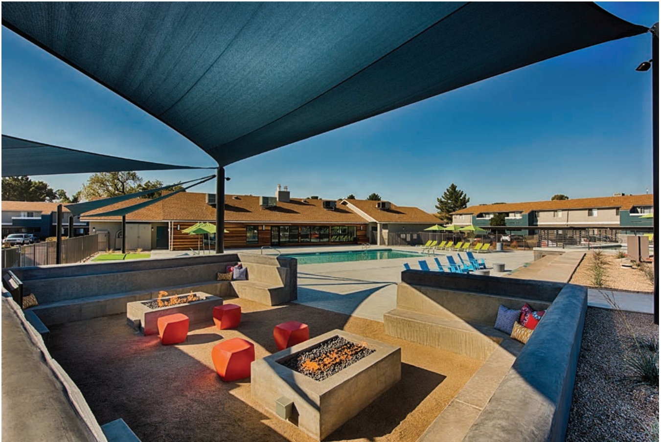
Indian Springs Apartments in Mesa, Arizona. In conjunction with local utility providers, Stratford Partners installed 2,652 CFL light bulbs, 600 water-reducing toilet tank banks, 1,060 faucet aerators and 600 low-flow showerheads at the property.
